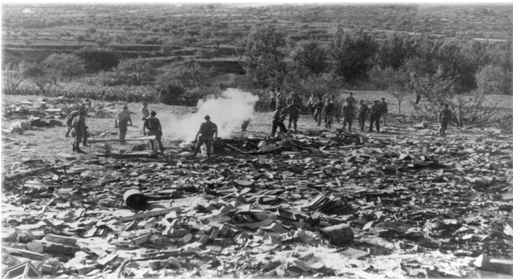
Here we can see the industry after the explosion.
